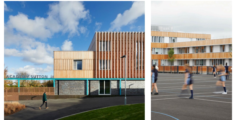
Harris Academy Sutton: a large secondary school built to Passivhaus standards (© Architype)
