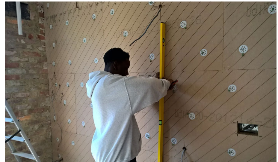
Installation of wood fibre insulation boards internally (Sources Back to Earth & ASBP)
