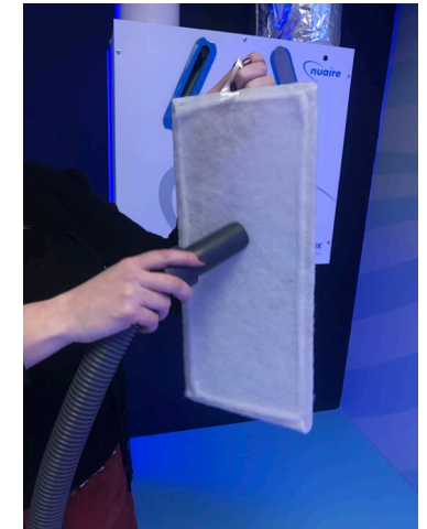
MVHR filters are easy to remove and clean, clean filters improve energy efficiency. (Sources: Vent Axia, Nuair.)
