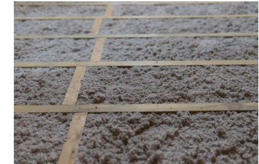
Cellulose- made from recycled paper (Source: Eco Spray Insulation)
