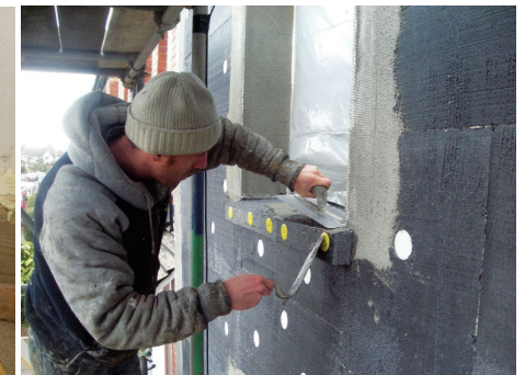
Photo of window install in Enerphit retrofit (Source: Passive House Plus)
