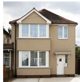
Grove Road, London (Source: Bere Architects)
