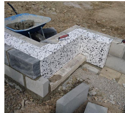
Left: an example of good Expanded Polystyrene insulation installation. Right: An example of poorly installed partial cavity installation, loosely fitting, and cement dropped atop and inside cavity (Source: Etude)
